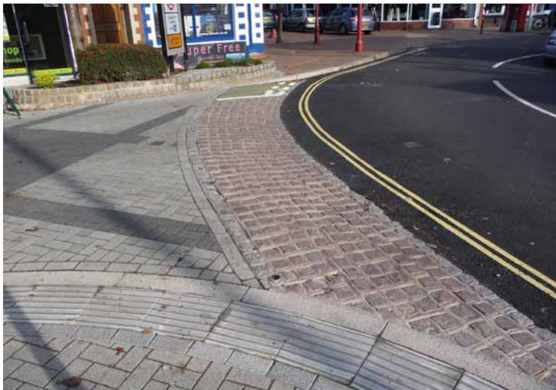
Figure 6.2 Example of a shared space gateway feature
